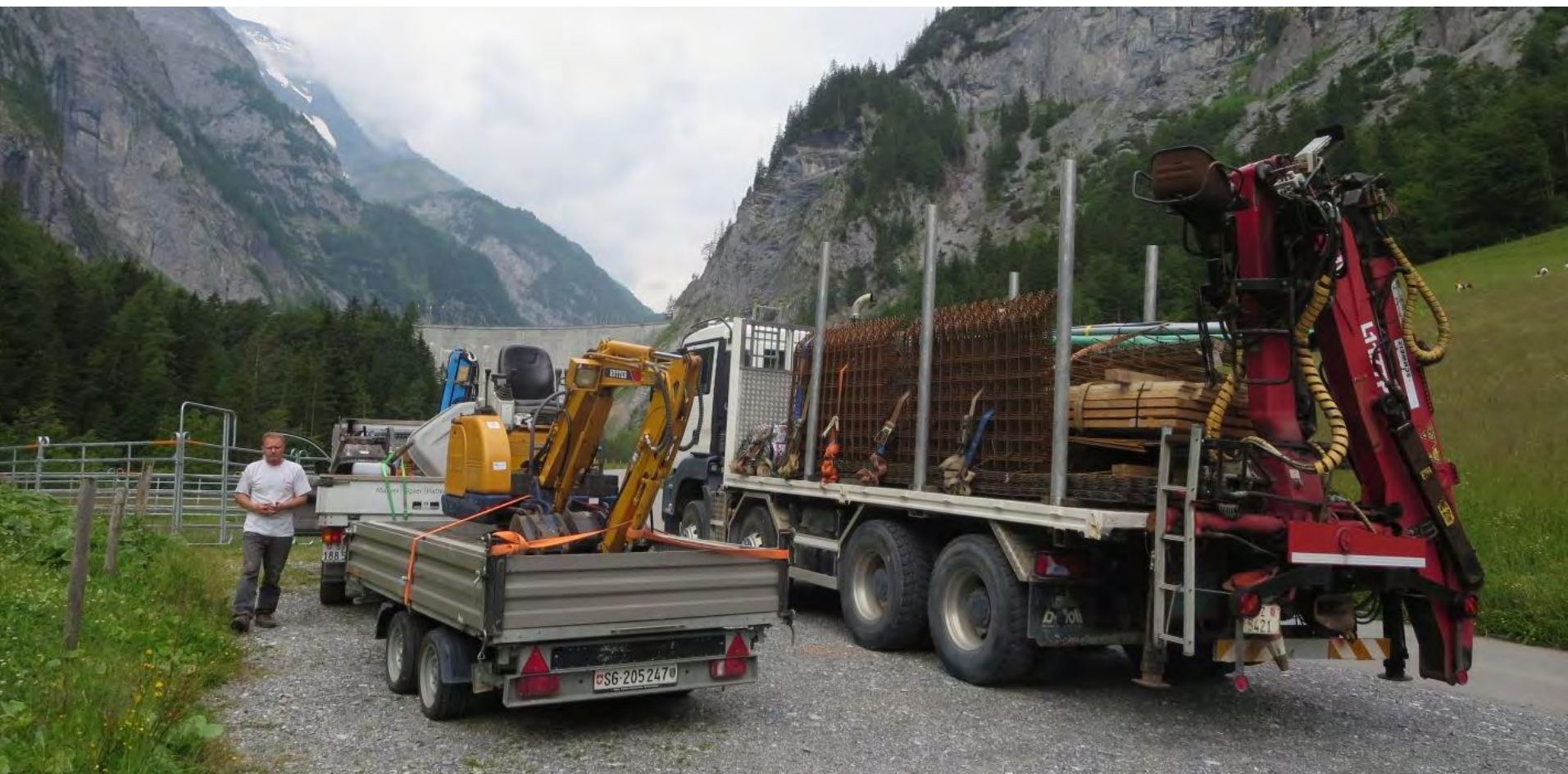
Transport Baumaterial zur Staumauer
